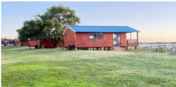
RENOVATED WOODEN COTAGES
