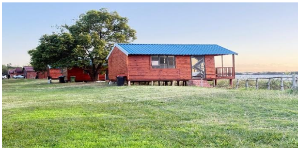
RENOVATED WOODEN COTAGES
