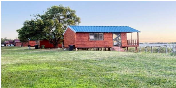
RENOVATED WOODEN COTAGES
